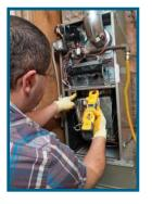
A tune-up can take up to an hour and a half to access the heat exchanger and determine whether or not the furnace is safe. A furnace may still heat your home but be unsafe to operate. If there is a safety issue, such as a crack in the heat exchanger, contact the manufacturer to see if it is under warranty.
